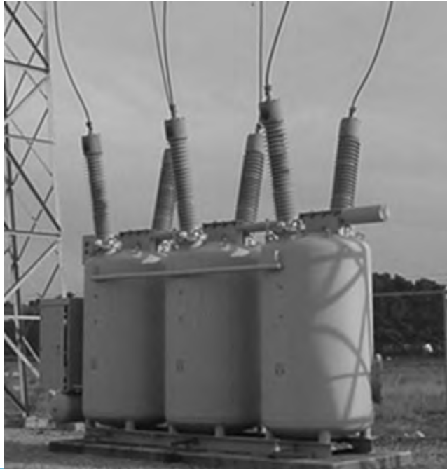
FIGURE 4.39 Three-tank bulk oil circuit breaker.
