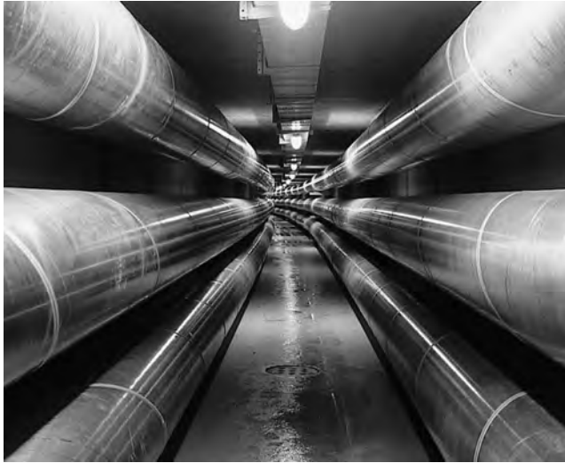
FIGURE 18.8 Tunnel-laid GIL for voltages up to 550 kV. (Courtesy of Siemens AG, Erlangen, Germany.)
