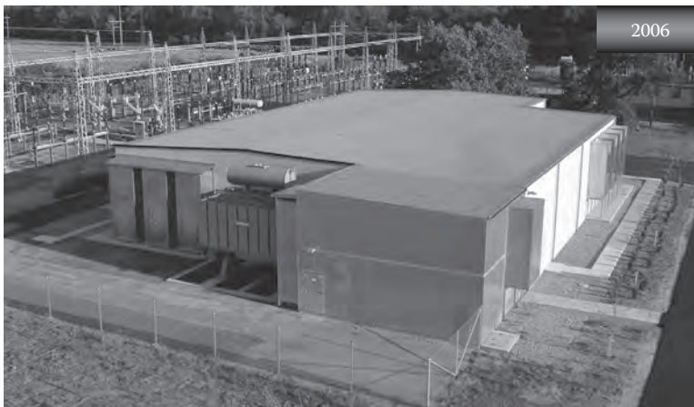
FIGURE 5.25 SVC Radsted: an innovative indoor solution for wind farm support—80 MVA r cap./65 MVA r ind., with extremely high requirements for noise abatement (upper part: single-line diagram; lower part: view of the substation).
