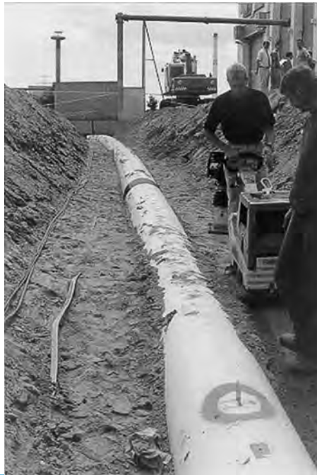
FIGURE 18.6 Bended tube and backfilling. (Courtesy of Siemens AG, Erlangen, Germany.)
