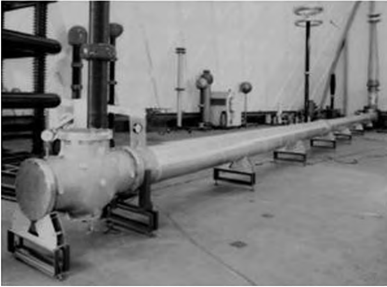
FIGURE 18.13 Test setup for high-voltage tests. (Courtesy of Siemens AG, Erlangen, Germany.)
