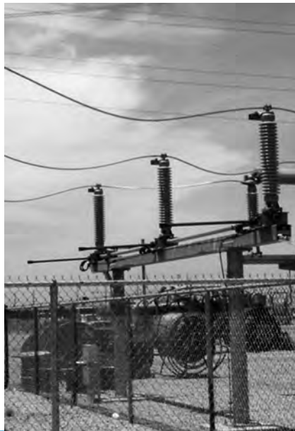
FIGURE 4.17 Vertical reach (pantograph) disconnect switch.
