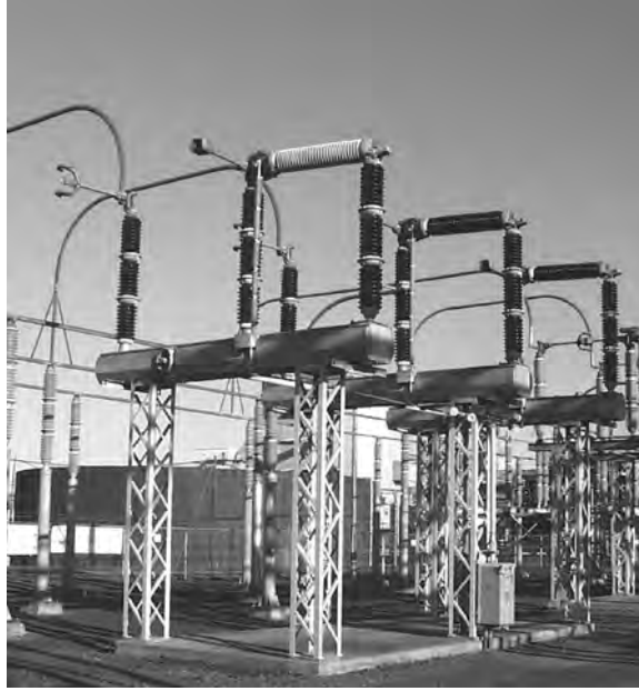
FIGURE 4.33 Multiple interrupter gap per phase circuit switcher.
