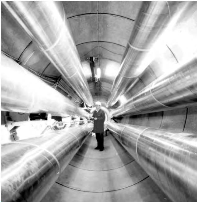
FIGURE 18.7 View into the tunnel. (Courtesy of Siemens AG, Erlangen, Germany.)
