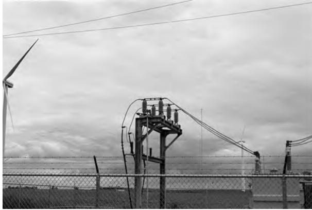
FIGURE 4.16 Single side break disconnect switch.
