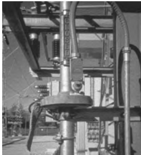
FIGURE 4.1 Mechanical cam-action type interlock.
