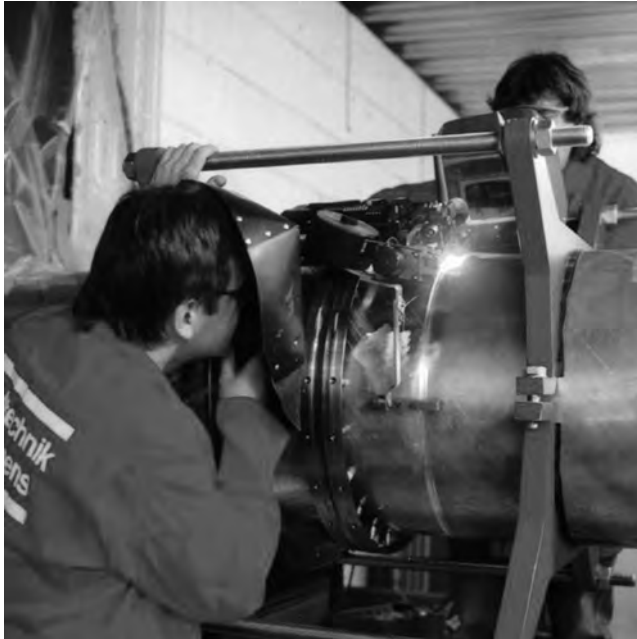
FIGURE 18.17 Computer-controlled orbital welding on site. (Courtesy of Siemens AG, Erlangen, Germany.)
