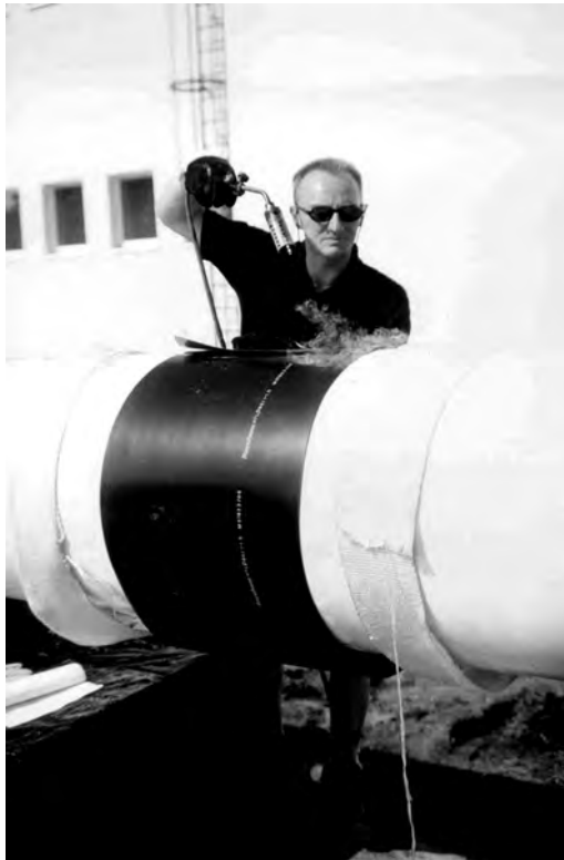
FIGURE 18.30 On-site corrosion protection of the welding area—shrinking method. (Courtesy of Siemens AG, Erlangen, Germany.)
