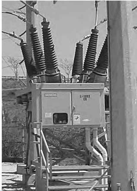
FIGURE 4.41 SF 6 gas dead tank circuit breaker.
