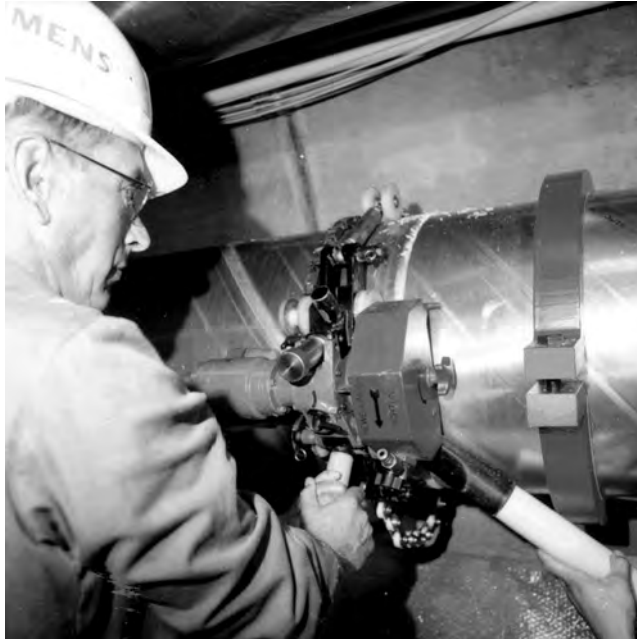
FIGURE 18.18 Cutting the enclosure pipe with a saw. (Courtesy of Siemens AG, Erlangen, Germany.)
