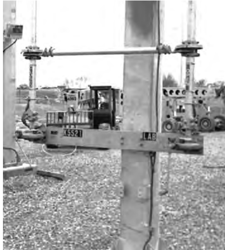
FIGURE 4.1 Mechanical cam-action type interlock.
